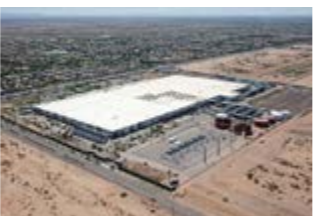
Aerial view of the Apple Data Center in Mesa near Phoenix, Arizona, US on August 6, 2017.
